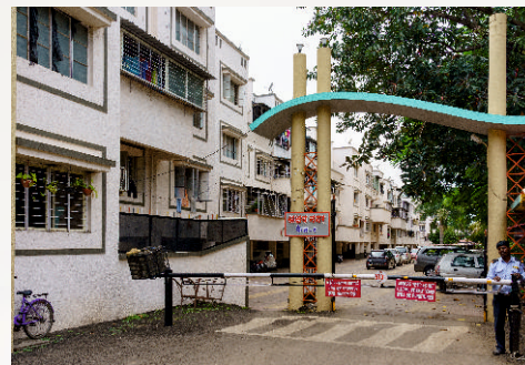
Akshay Nagar Phase I Pimple Nilakh, Pune NO. OF FLATS : 112
